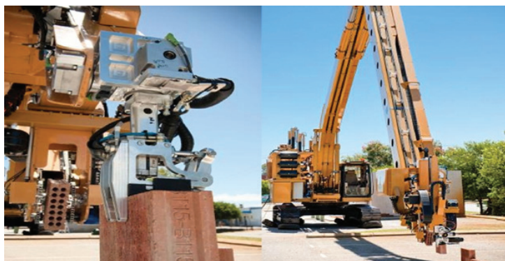
Figure 3 – 3D house construction with robots.
